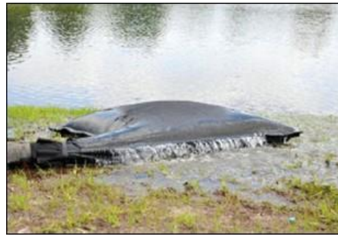
Plate 2-2 Silt Bag with water being pumped through
