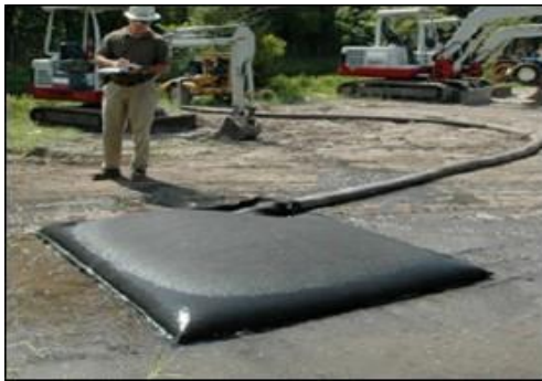
Plate 2-1 Silt Bag under inspection
